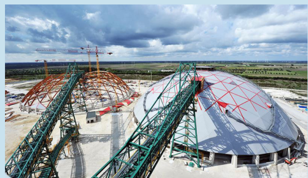
Figure 2: Conveyer belt towards the dome
