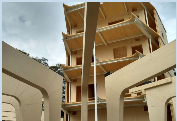
Figure 1: Timber cantilever rafters and core
