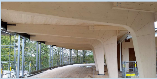
Figure 2: Standard floor with timber rafters
