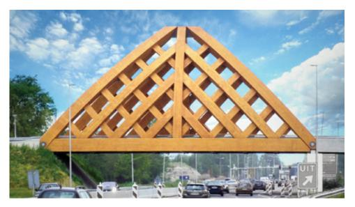
Sporting a solid, complex shell construction made from exposed wood beams, a bridge located in the Netherlands was designed to reference the town of Sneek's historical water gate landmark.
