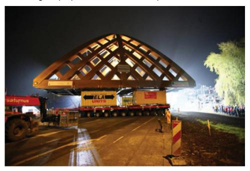
Two self-propelled modular transporters (SPMT) vehicles were used to move the 400-ton bridge 2,624 feet, 8 inches from the assemble area to the final location.
