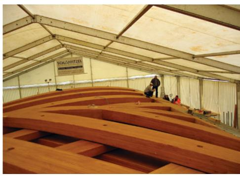
To prepare for final assembly, workers placed a large tent over the shells and heated it. After this, the bonding of the threaded rods using the prepared holes could take place.
